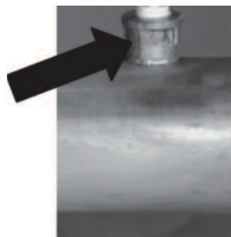
Fig. 22: Installation with Weld O Lets
